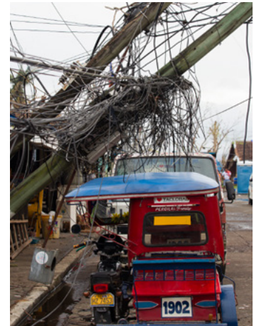
Much of the existing telecommunications infrastructure in Tacloban, Philippines was shredded by Typhoon Haiyan. A UMNS photo by Mike DuBose
